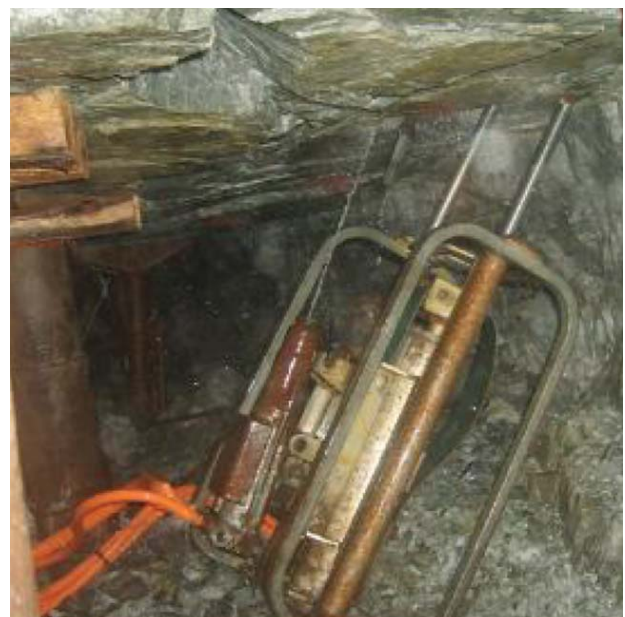
Figure 15—Drilling of support holes @ 70° towards the stope face, at a deep-level gold mine in the West Rand, in very bad ground conditions
